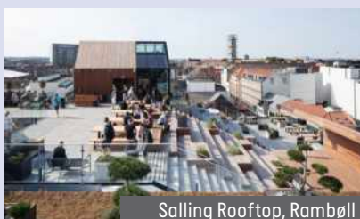
Salling Rooftop, Rambøll
